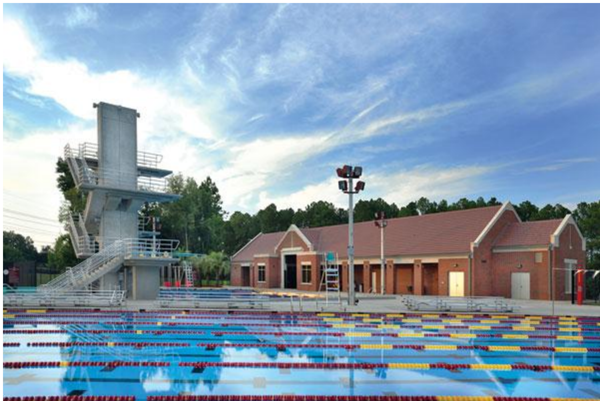
Figure 2: FSU Morcom Aquatics Center
