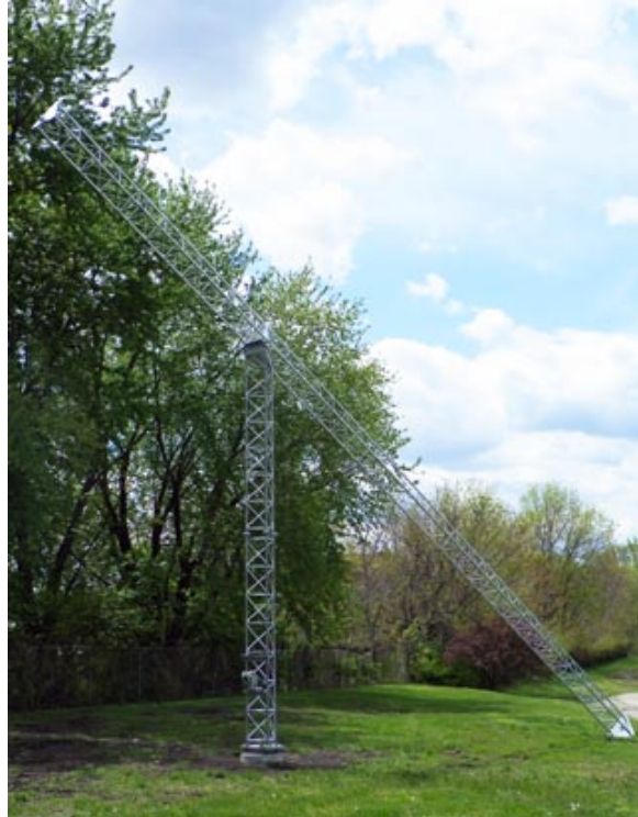
Figure 5.1.1 – Illustration of Self Erecting Tower
