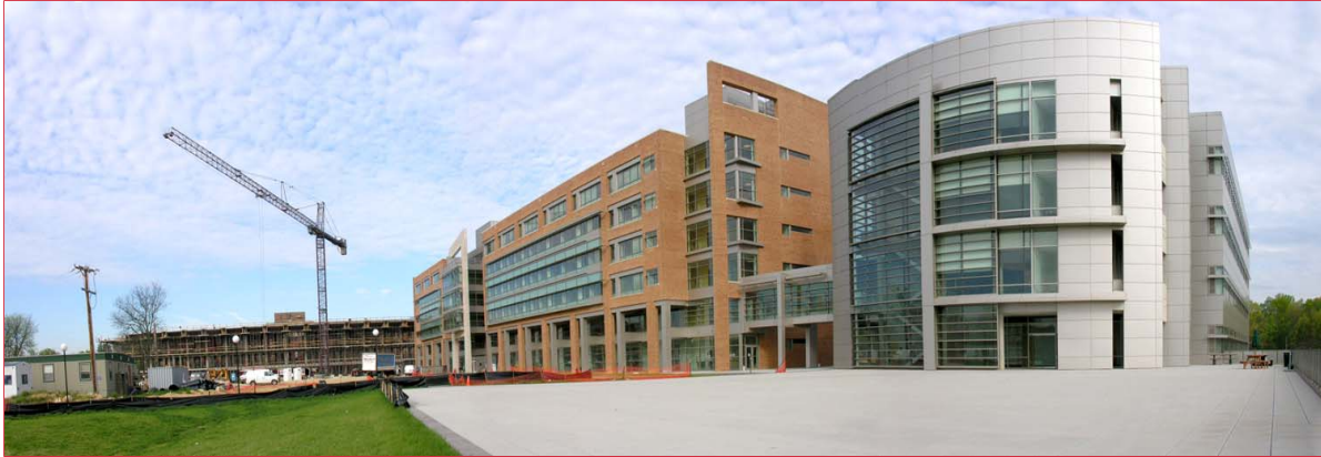
FDA Consolidation (CDER and CDRH Life Sciences Laboratory/CDER Office Building) | White Oak, MD
