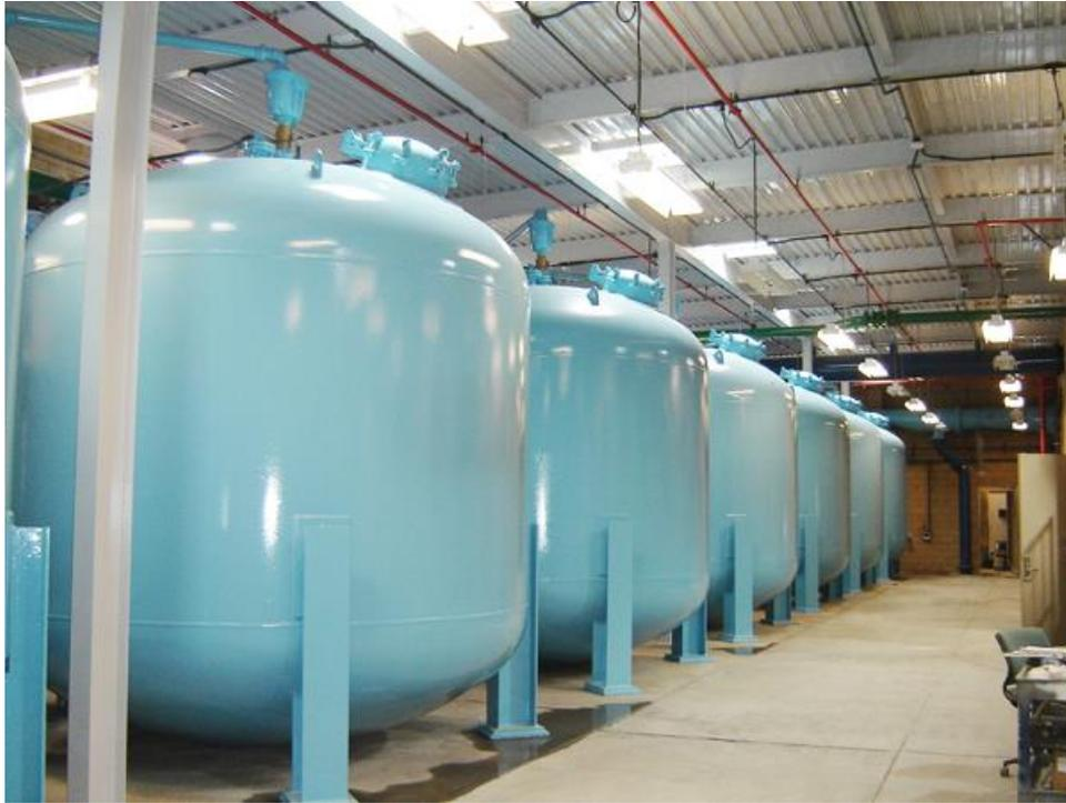
**Figure 9. Pressurized Filters for Large-Quantity Treatment**
