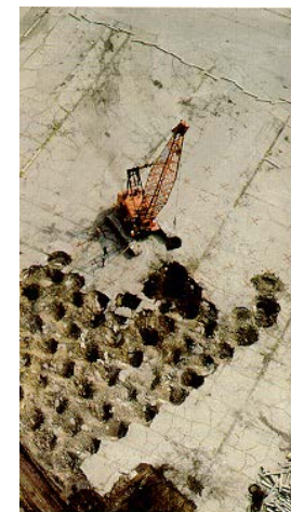
6- Dynamic Compaction
