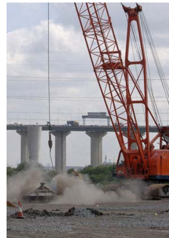
6- Dynamic Compaction
