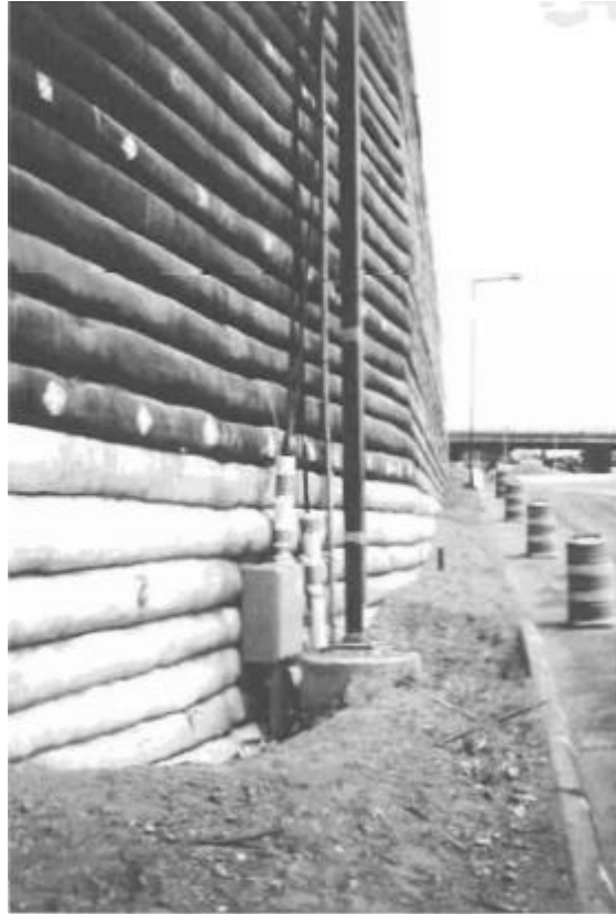
Fig. 2.4: A completed Wrapped-Faced GRS wall (courtesy Washington Department of Transportation)
