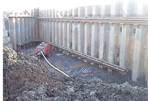
Sheet pile wall
