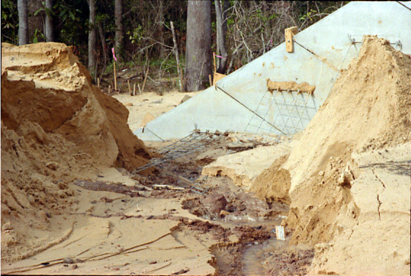
Mechanically Stabilized Earth Wall (MSE Wall)
