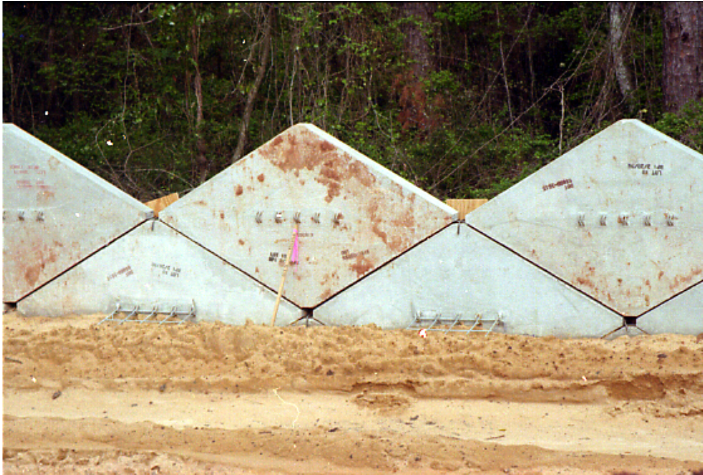
Mechanically Stabilized Earth Wall (MSE Wall)
