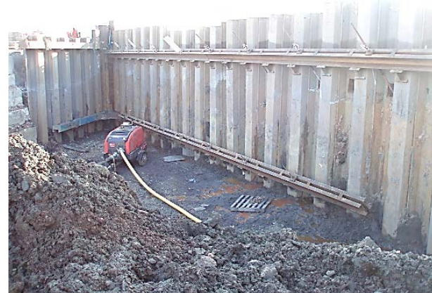
Sheet pile wall
