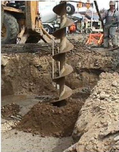
First the auger drills deep into the ground.
