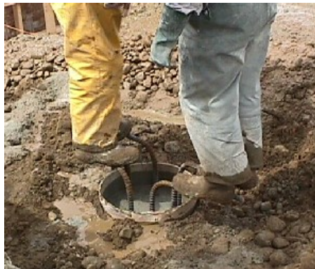
One last push to get the steel all the way in.
