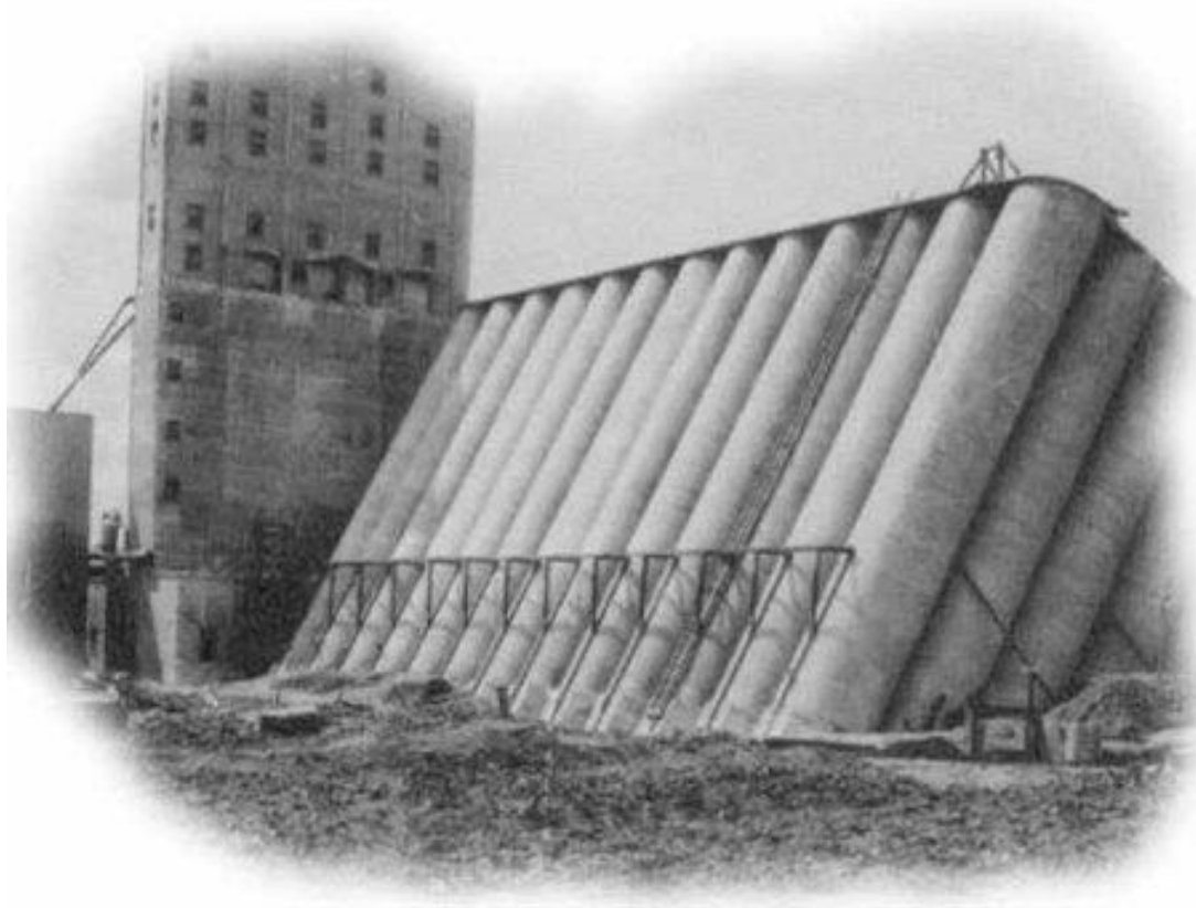
Bearing Capacity Failure
