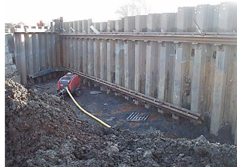
Sheet pile wall
