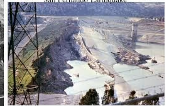
Failure of Van Norman Dam from 1971 San Fernando Earthquake
