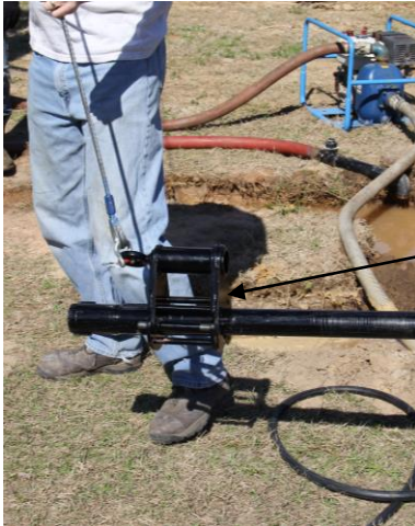
Figure 11 (Folder: LS_New Rig) (LS_New Rig 181.JPG)
